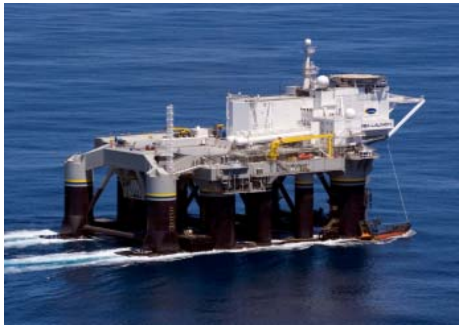
The Odyssey Launch Platform enroute to the equatorial launch site at 154 degrees West Longitude (Source: Sea Launch)
